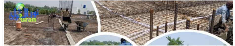
Alhamdulillah 28 th July 2024 Final Third floor roof done in MASJID NURULQURAN
